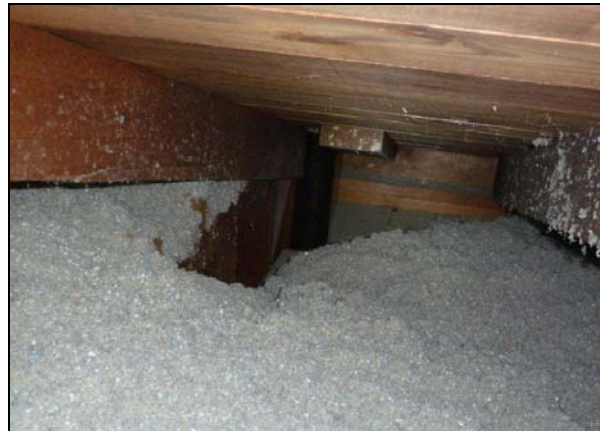
Missing insulation
