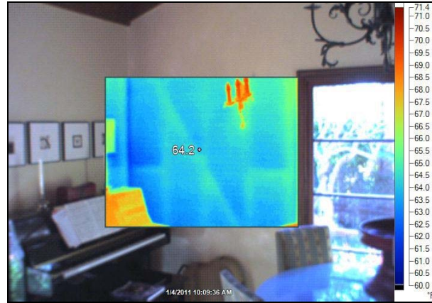
Note studs and bracing
